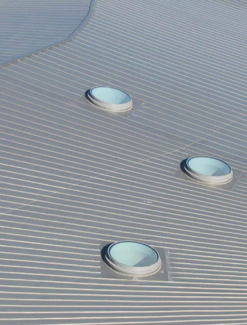
“ Each sheet was individually rolled and shaped so that all seams pointed to two control points on either side of the pool. ”
